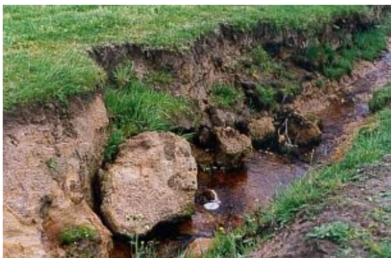
Figure 2. Open drain with incorrect bank matter.
