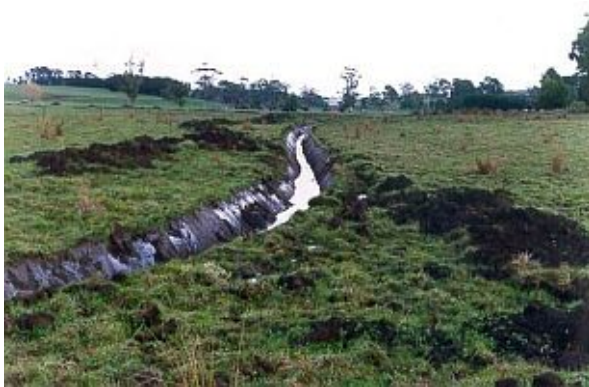
Figure 1. Medium sized "V" shaped open drain.
